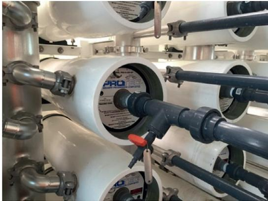
each stage is monitored, and performance can be calculated and/or normalized to a set of standard conditions. Permeate conductivity from individual pressure vessels or membrane elements can also be used to isolate performance and initiate corrective measures. Thus, three of the criteria of an IVP—continuous indirect integrity monitoring, diagnostic testing and membrane repair, and replacement practices—exist within existing plant operations.
